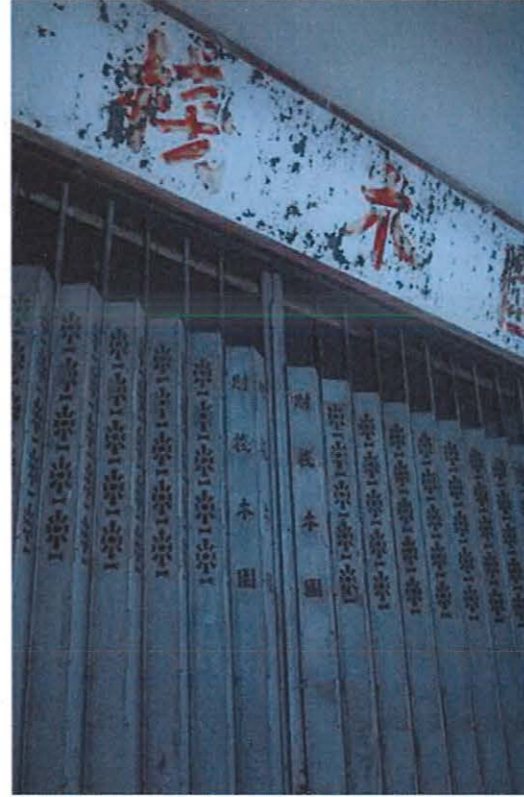
METAL SHUTTER OF A OLD SHOP.
