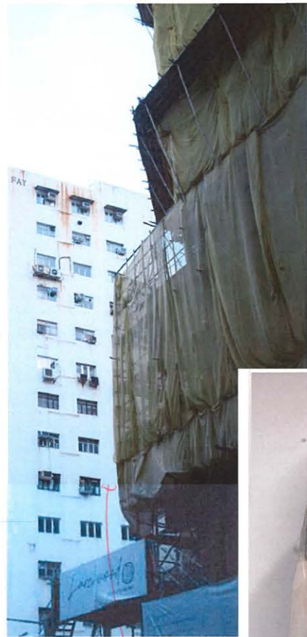
TRANSPARENT FABRIC ON SCAFFOLDING.
